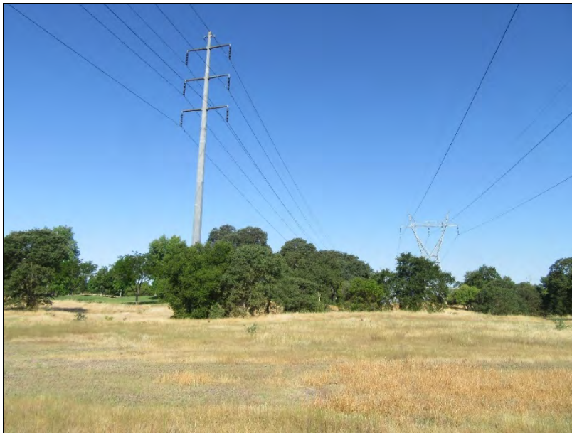
Figure 5. Transmission lines within central portion of APE (view west; June 23, 2020).
